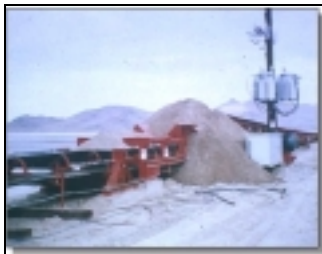
Figure 3, Plugging and Spillage.
