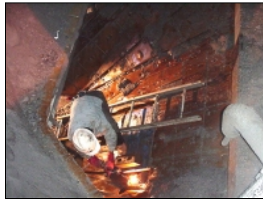
Figure 27, BC400 Chute Inside, looking down from the top.
