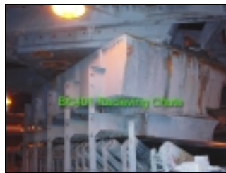
Figure 15, Back Iso Receiving Chute
